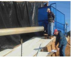
Hopper With Outlet Pipe Leading To Area Inlet
